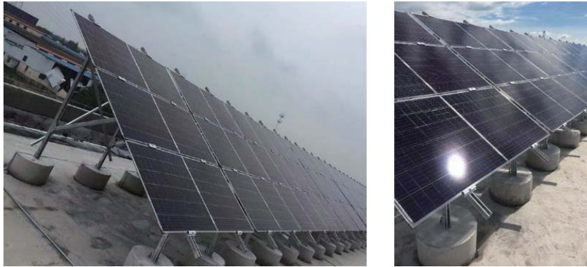
Figure 3 Picture of Haining cement project
